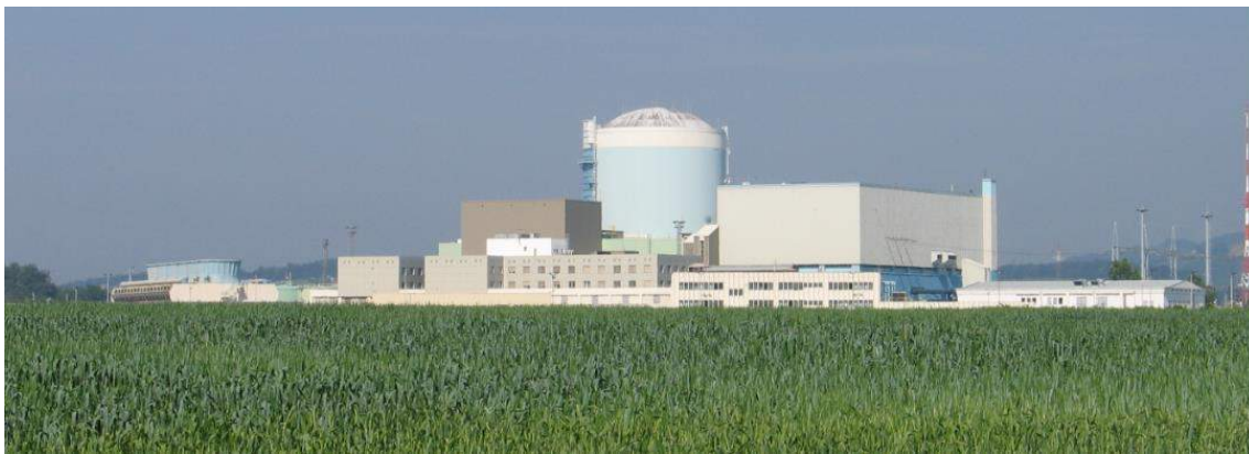
Figure 91: View of NEK from the southeast (source: /193/)
