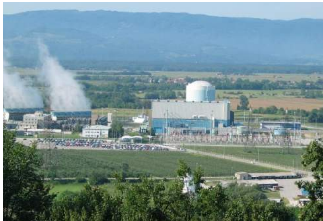
Figure 87: Visible plume from NEK's cooling towers (source: /116/)
