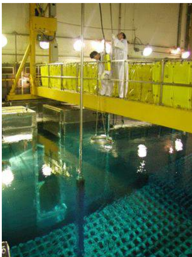
Figure 69: Insertion of a spent fuel element in a rack in the spent fuel pool /233/
